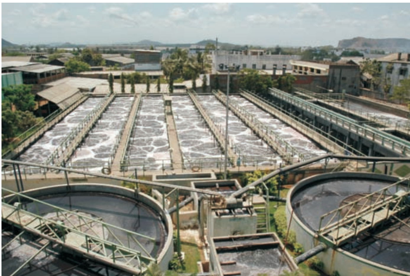
A common effluent treatment plant at Chennai
